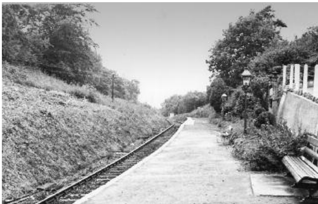
Wootton station looking west in 1949. The bank on the left was unstable then.
