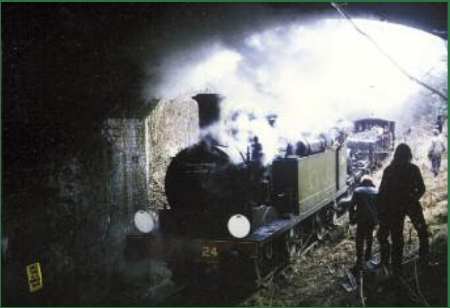
W24 proceeds gingerly over distorted trackwork and under Station Road bridge, Wootton, with a selection of goods wagons.
