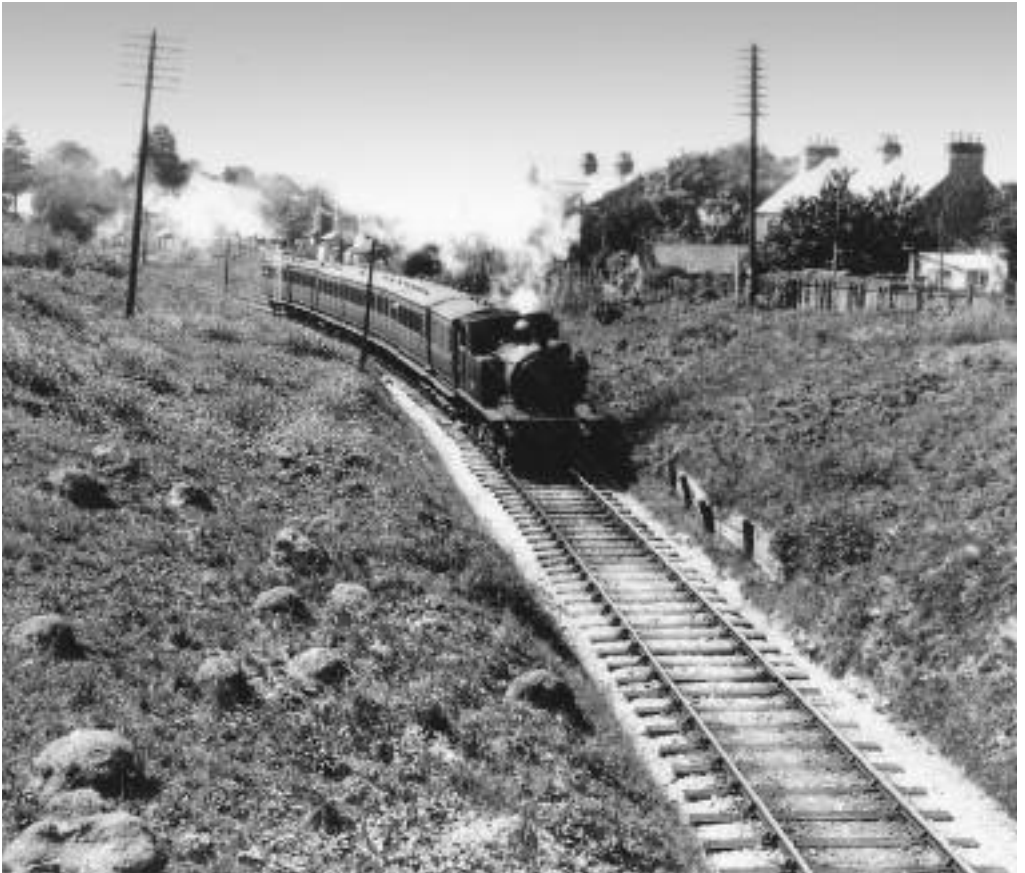
Looking south from Cross St bridge, an unidentified O2 has just passed Newport down distant from Ryde signal with a Ryde-bound train about 1930. Photo: A.B.MacLeod
