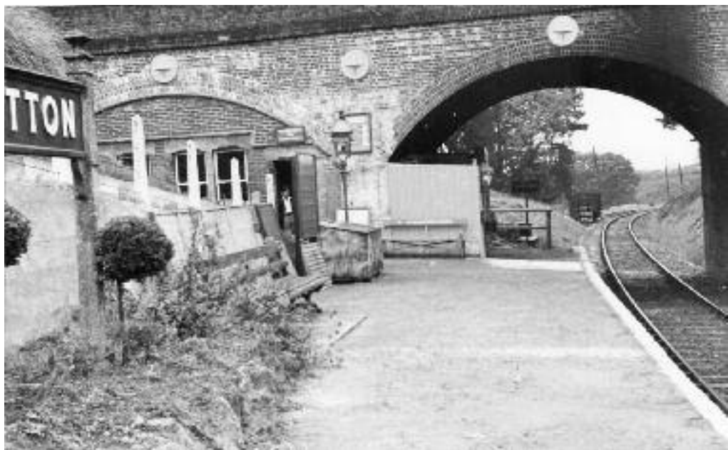
Wootton Station looking east. The station offices were situated in one of the bridge arches and a solitary coal wagon stands in Charlie Osborn's siding. 1949.
