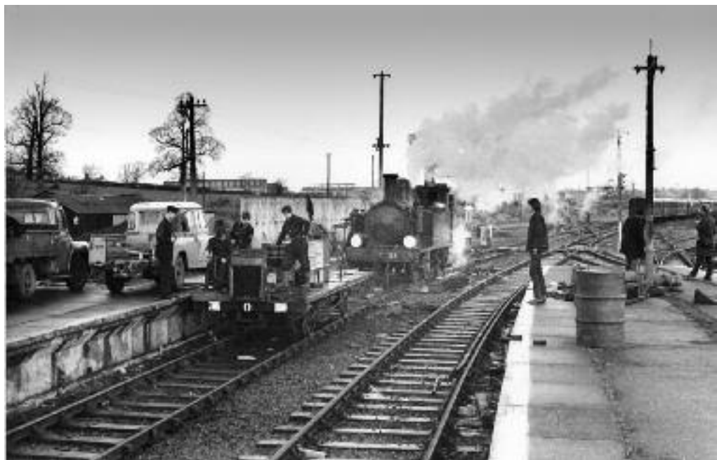
The chassis of the Ryde Pier Tram is prepared for a test run to Havenstreet. Photo: Gary Merrin.
